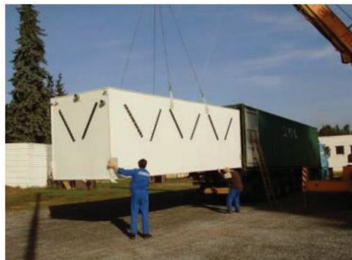
Fig. 3 Transportation of a container water treatment facility [5]
