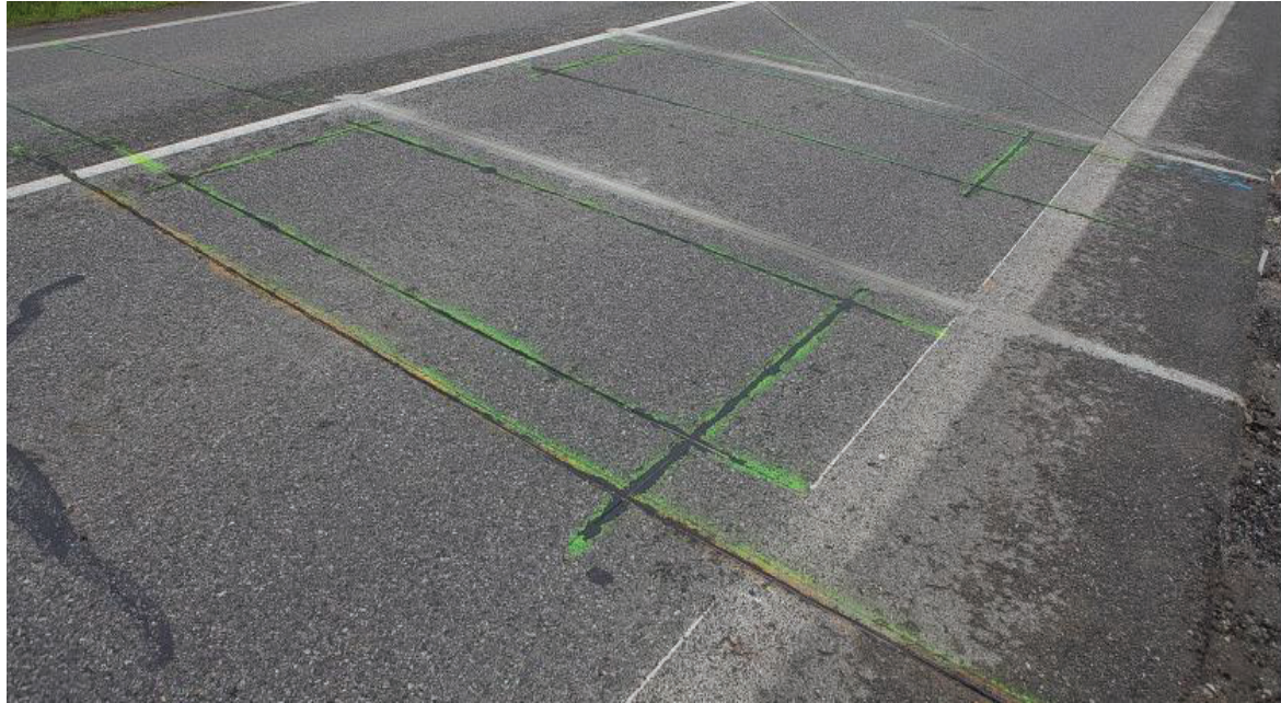
Fig. 4 Piezoelectric detectors combined with induction loops [5]
